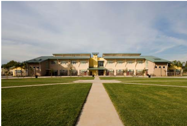
New Two-Story Classroom Addition Cajon Valley Middle
